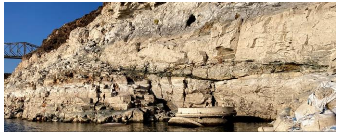
Drinking water Intake No.1 is visible above the surface of shrunken Mead reservoir which provides nearly all of Las Vegas’ water. Photo courtesy Southern NV Water Authority
